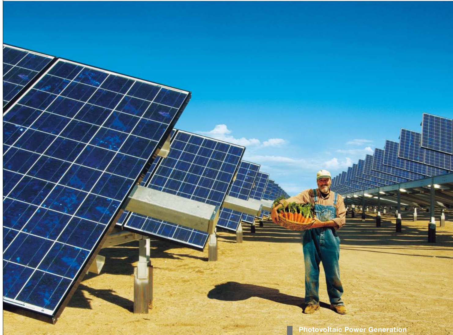
Bolthouse Farms, Lancaster, California, USA. System size: 1.9 MW
